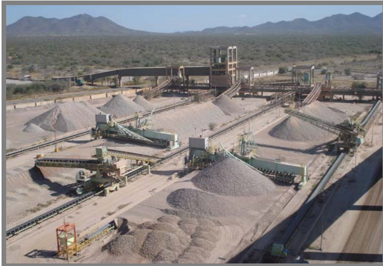
Limestone Handling System – Yaqui Plant - Cemex (Mexico)
