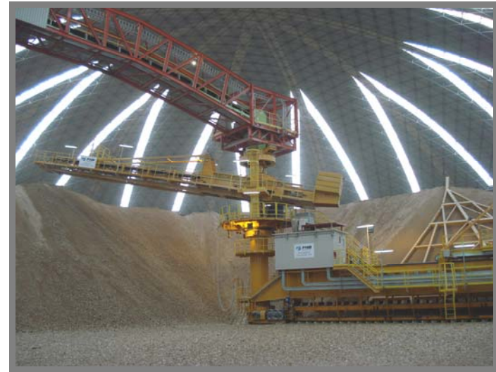
Limestone Circular Stockyard – Merida Plant - Cemex (Mexico)
